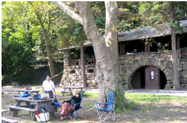
The Alpine Boat Basin Pavilion
